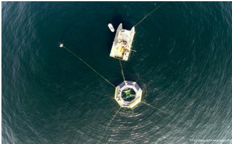
Figure 24 – Seatricity's Oceanus 2 device being installed at Wave Hub in summer 2014 by the Ocean Enterprise
