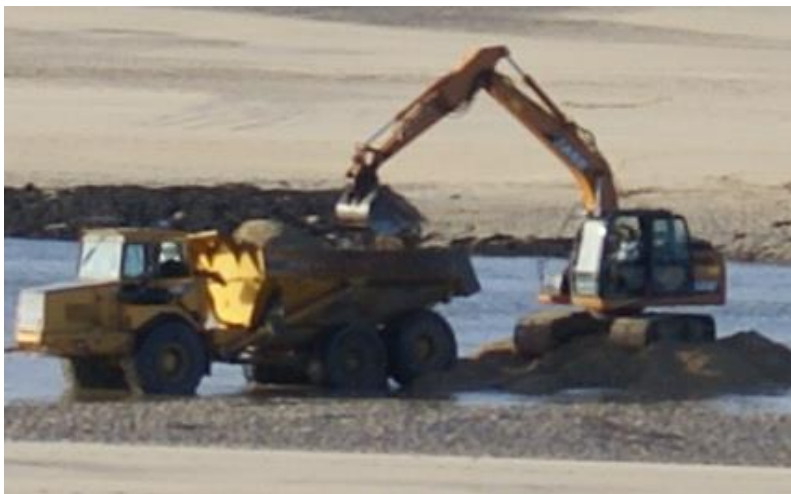
Figure 18 (left) – mechanical dredging in the Hayle access channel in 2010.
